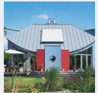
Private Residence, Bad Iburg Germany
